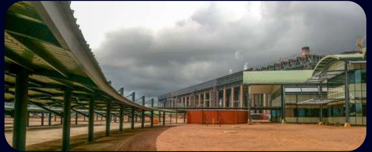
ESKOM - Design of most of the non-power island infrastructure at Medupi and Kusile Power Stations
