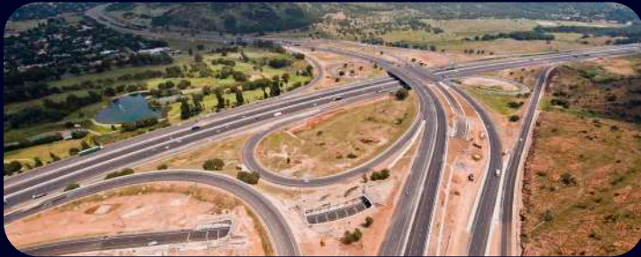
South African National Roads Agency Ltd (SANRAL) - Upgrading of N12 Section 18
