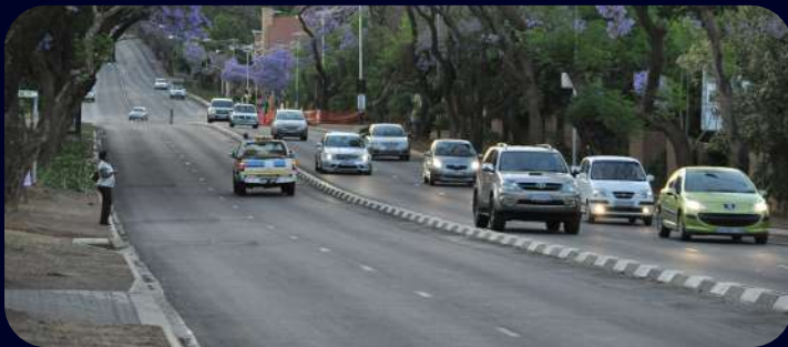
City of Tshwane - Upgrading of Charles Street, Pretorius, Schoeman, Duncan and the Hatfield one-way system
