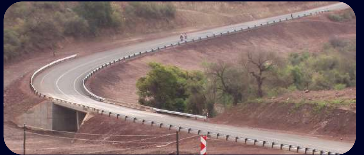
Roads Agency Limpopo (RAL) - Upgrading of Section of Route D4050/D1583 between Mafefe and Sekororo
