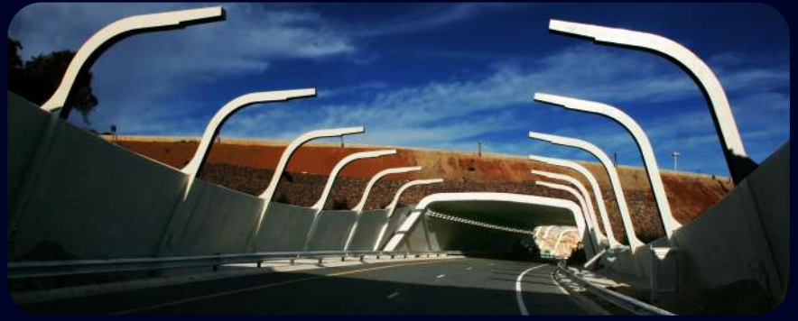
South African National Roads Agency (SANRAL) - Reading Interchange Cut & Cover Tunnel
