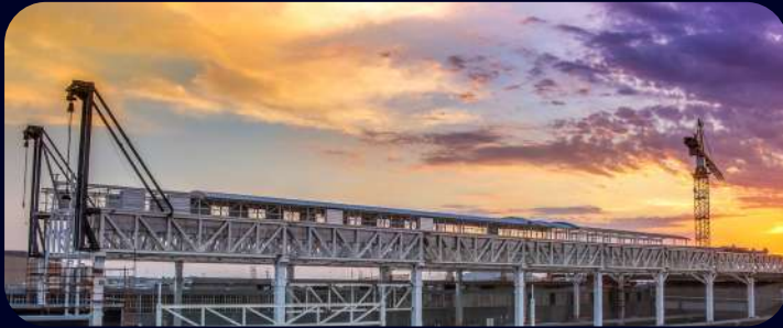
BMW South Africa: Building 50.0 - Assembly Plant Roof Lift (SAICE 2017 Structural Steel Award & Overall Most Outstanding Civil Engineering Project)
