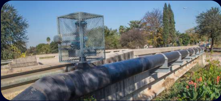
City of Tshwane - Design and construction monitoring Gezina Bulk Water Pipeline
